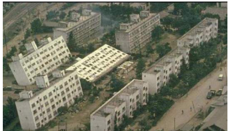
Figure 52 Soil liquefaction
